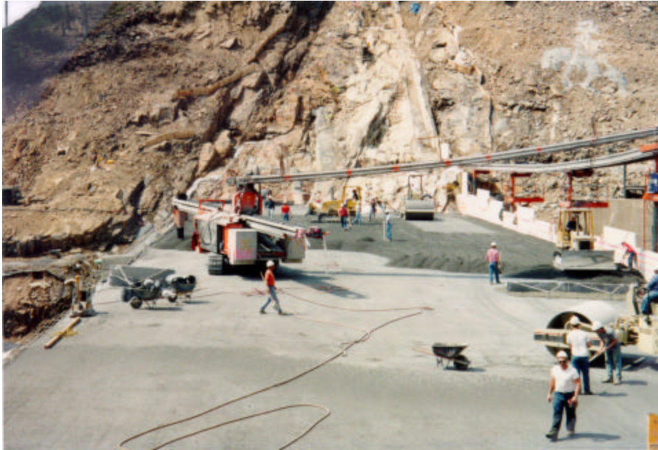
Figure 6-1. Conveyor system with self-propelled crawler-placer
