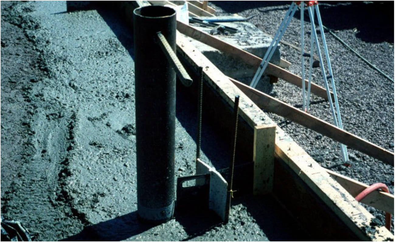
Figure 6-5. Installation of waterstop, joint drain, and crack initiator
